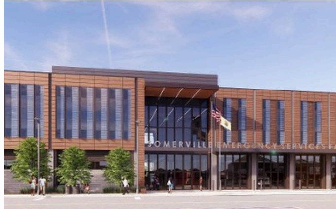
EMERGENCY SERVICES FACILITY
